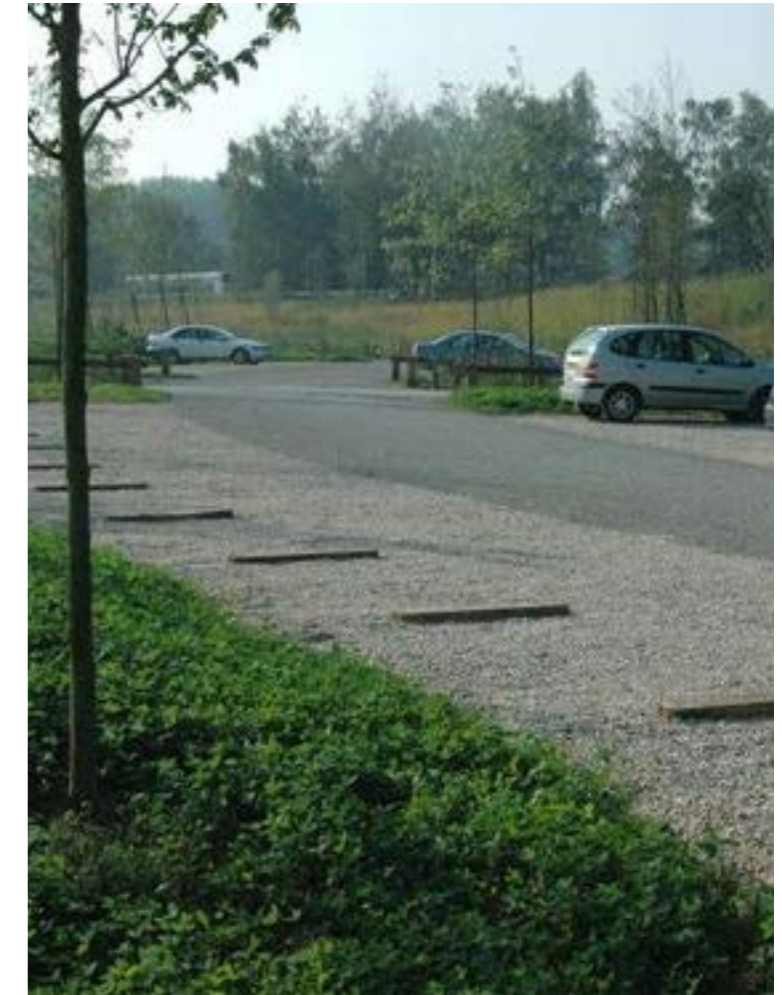
Clearly marked parking bays to maximise the efficiency of the car park. Logs or a similar natural material appropriate to the location to be used to mark out parking bays.
