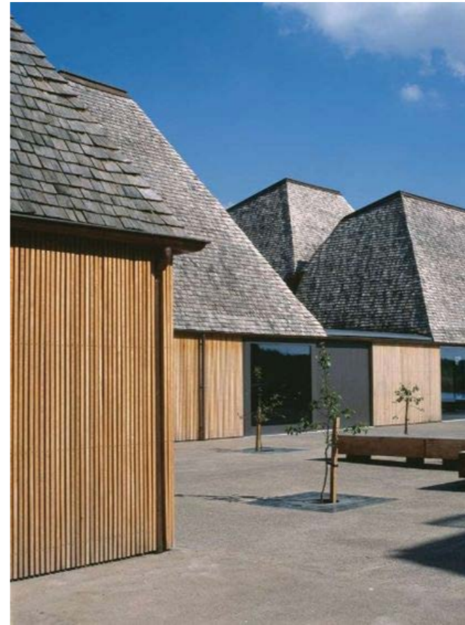
Example Image: 3. Naturally weathered timber shingle roof and simple dark framed glazing
