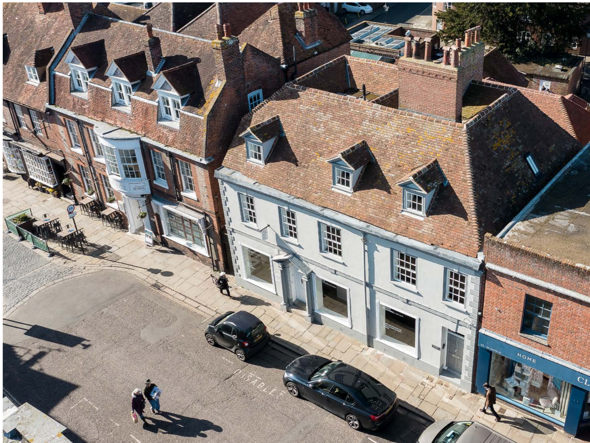
Photograph - 32 North Street, Chichester
